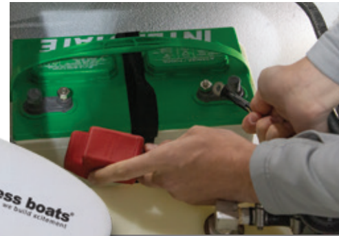
Install marine batteries
